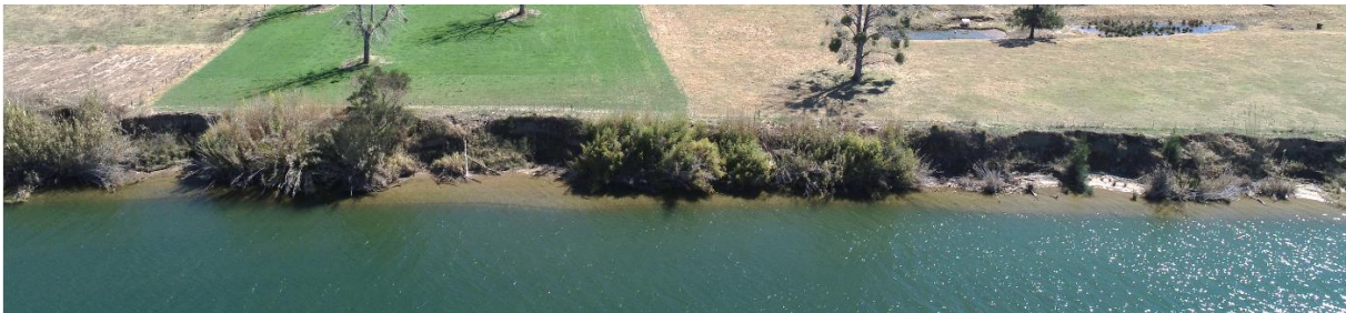
Figure 1. Example of eroding riverbank without bank protection
