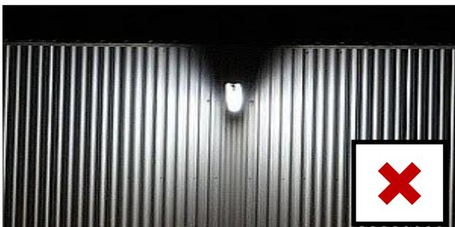
This double fluoro has no shielding emitting light sideways and upwards
