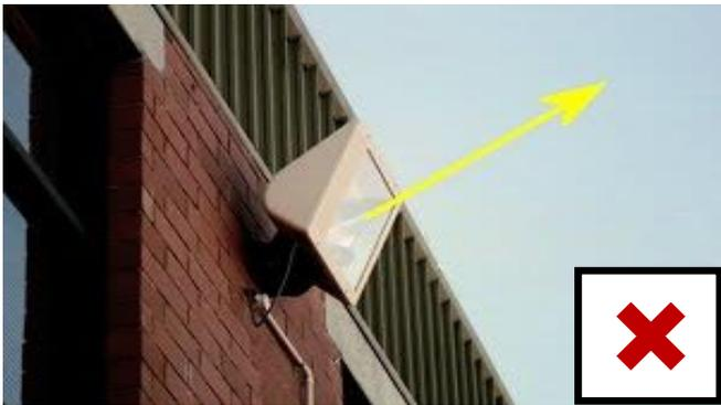
This light is incorrectly aimed so most light is wastefully beamed into the sky
