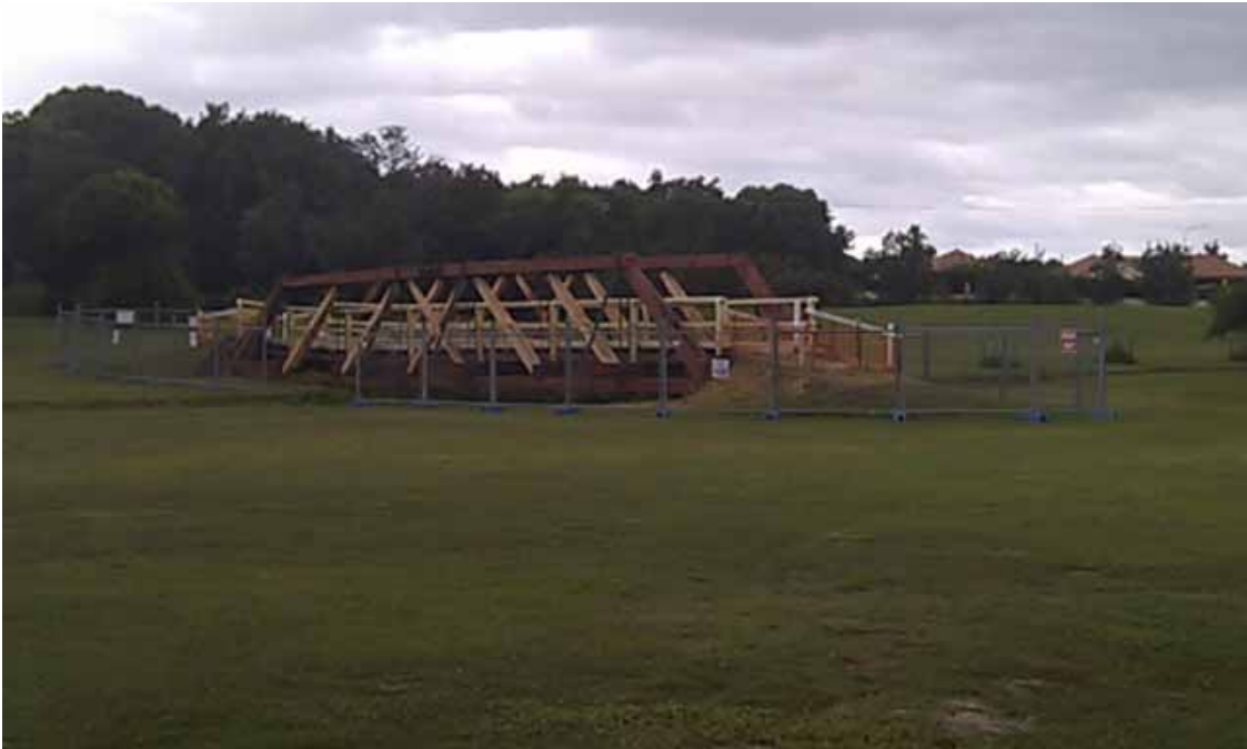
Figure 1 – Fenced Story Bridge
