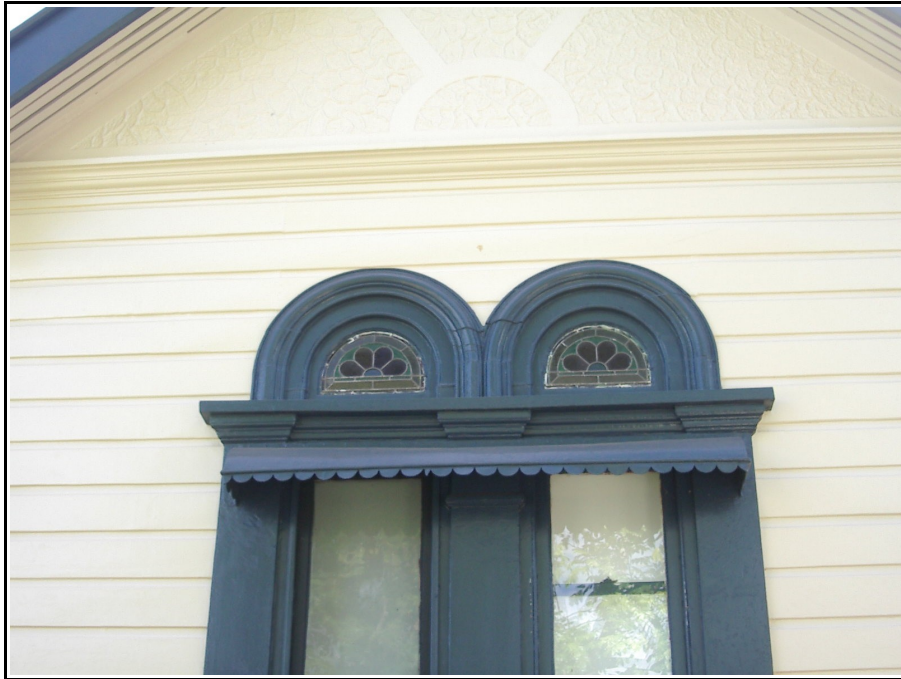
Figure 3.12 Window Mouldings, Pound Street
