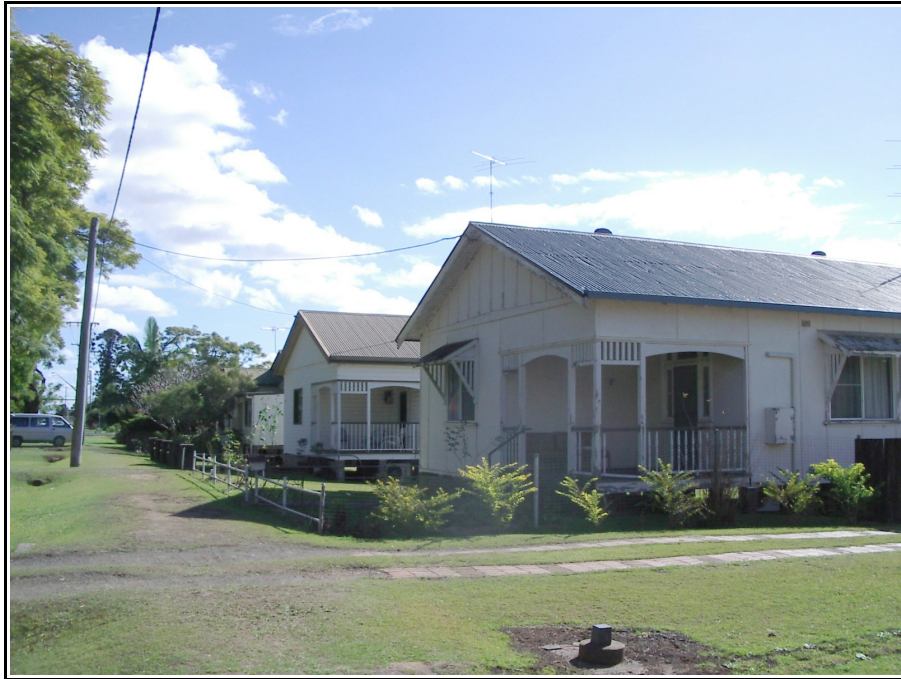
Figure 3.17 Cement Sheet Cladding, Pound Street Group
