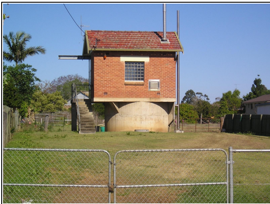
Figure 3.21 Sewerage Pump Station, c1930
