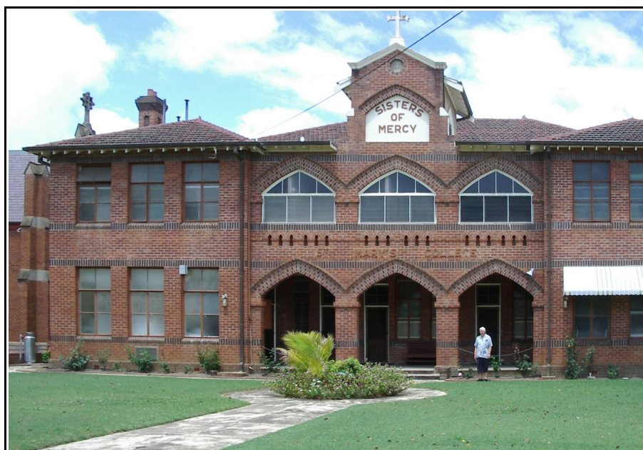
Figure 3.19 St Mary's College - St Marys' Precinct
