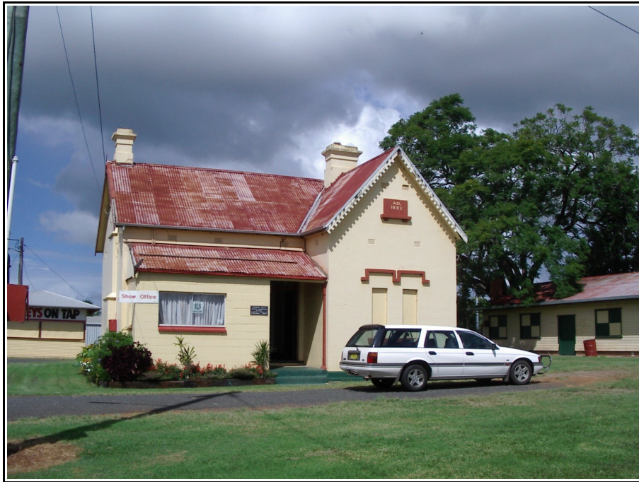
Figure 3.5 Caretakers' Cottage, Showground
