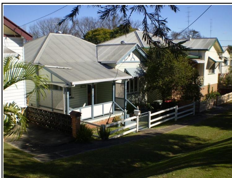
Figure 4.5 Cottage, Spring Street, South Grafton
