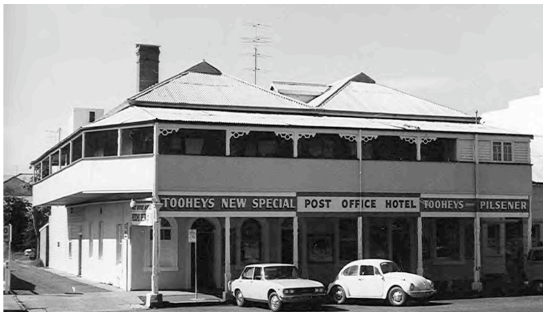
Figure 2.9 Post Office Hotel, Victoria Street, 1973 ( source : National Trust of Australia)
