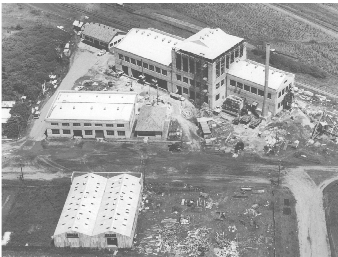
Figure 4.1 Peters Dairy Factory under construction, c. 1953. The small building at the left rear is the company's depot, in operation by 1951. (Source: Roger Harrison, Grafton)
