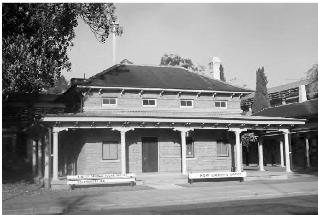
Figure 2.2 Former Grafton Court House, 2007. This structure is the 1880s extension to the second (1861) court house, the ruins of which adjoin it at the rear. The sign erroneously states that this is the 'site of [the] original police station constructed 1847'.
