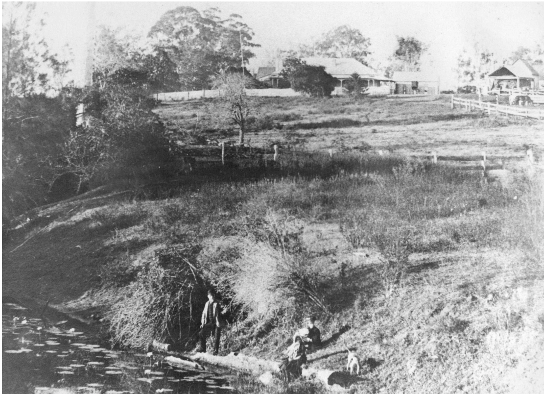
Figure 1.2 Small house in 19th century ( Source: Clarence River Historical Society)
