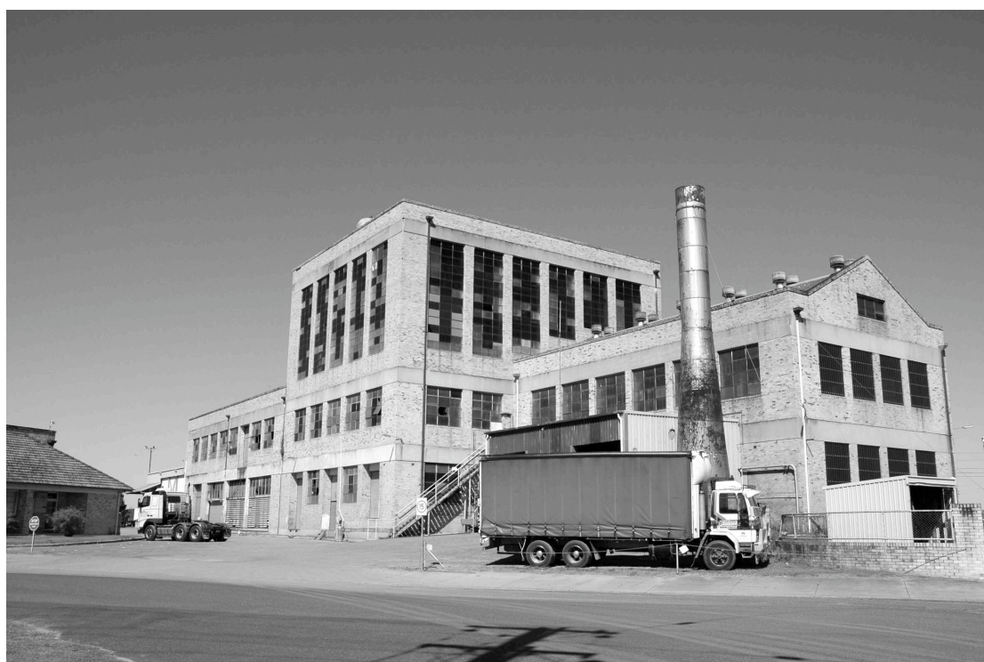
Figure 4.2 Former Peters Dairy Factory, 2007
