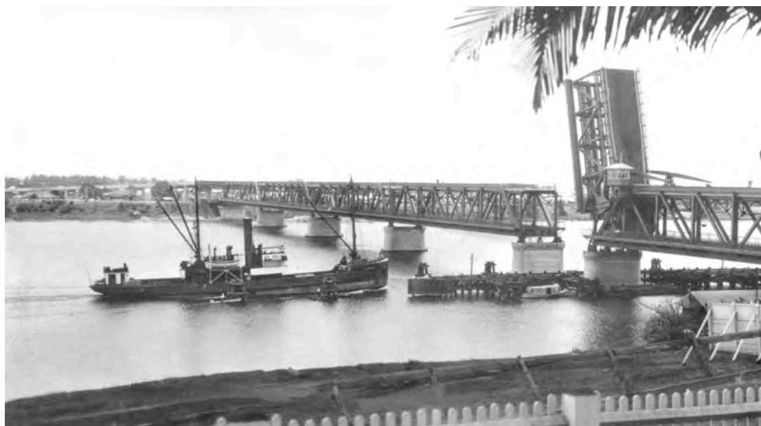
Figure 3.4 A view of the Clarence River bridge from South Grafton. The bridge was opened for rail and road traffic in 1932.
