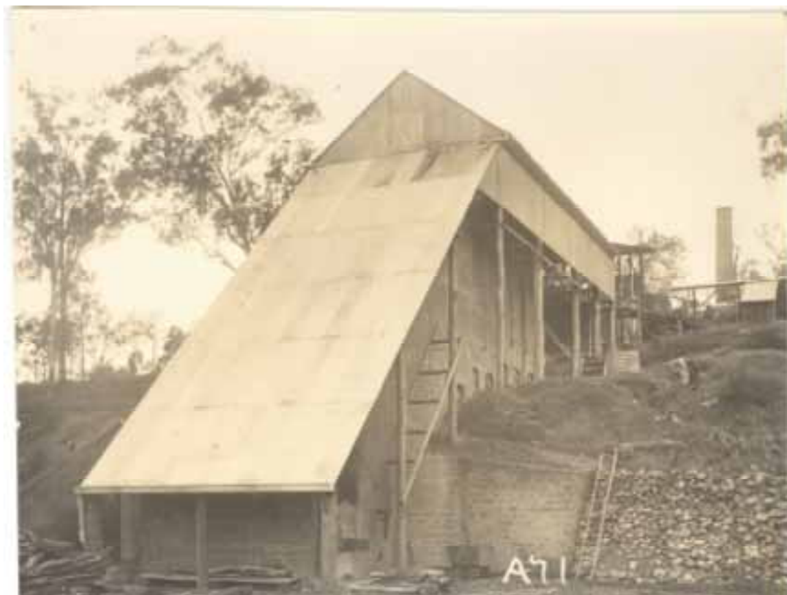
Figure 3: The second (c.1914) Pulganbar mercury smelter; view upslope from near Pulganbar Creek.
