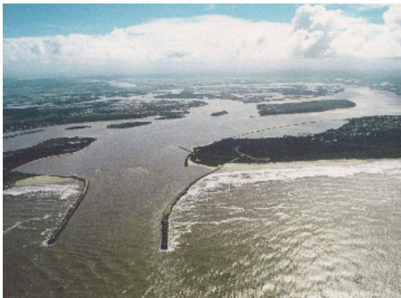
Photo 1: Clarence River Breakwalls
