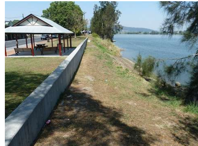
Levee walls protect both parks and reserves and communities at Grafton, Ulmarra and Maclean
