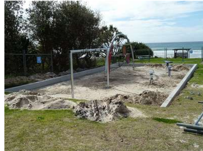
New playground being installed to encourage active play
