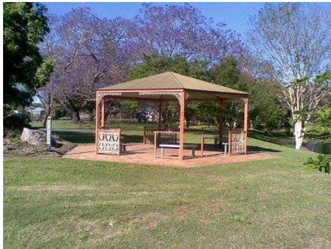
Council has an on-going responsibility to ensure park/reserve infrastructure is in a safe and serviceable condition
