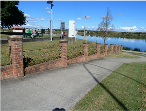
Boundary fence with Prince Street (below levee wall)
