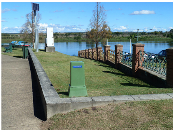
Masonry block levee wall adjoining Prince Street
