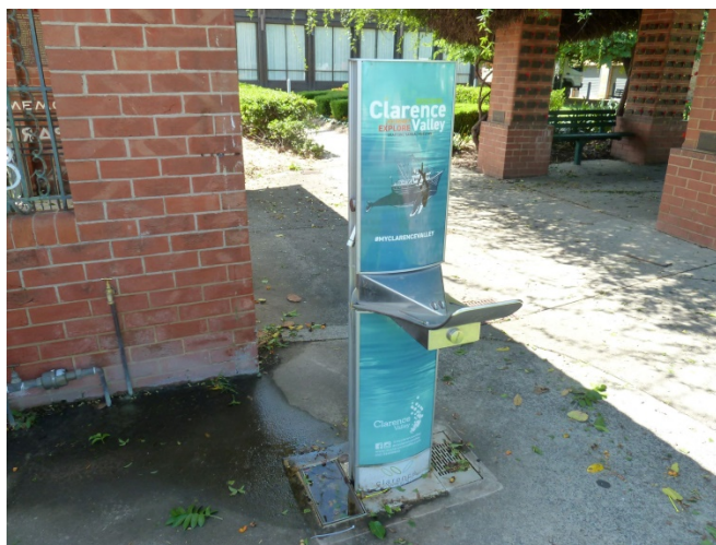
Figure 4.22: Water from drinking water fountain pools at base of entry gate brick work
