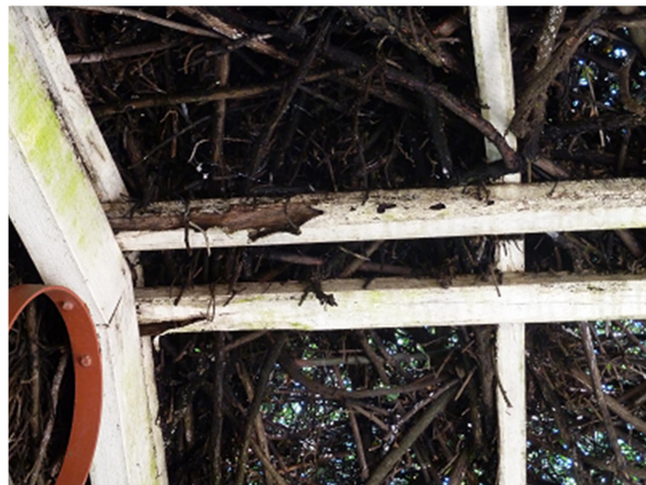
Rotting timber in Pergola near entry gate
