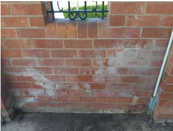
a. Rising damp on entry gate brickwork
