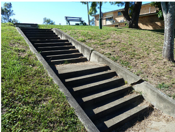
Concrete stairs showing cracking in side wall
