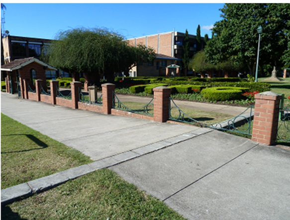
Boundary fence with Prince Street (above levee wall)
