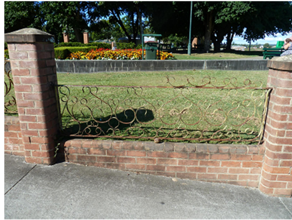
Rolled iron infill panel
