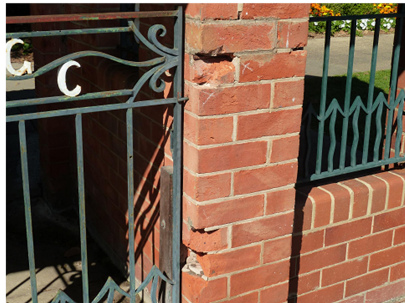
b. Damaged brickwork on entry gate
