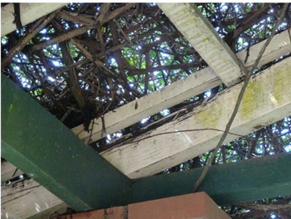
Rotting timber in Pergola near WWI memorial
