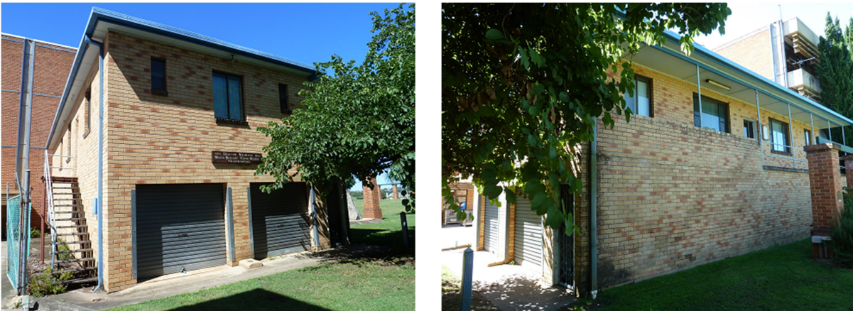
Figure 4.12: Grafton Water Brigade building
