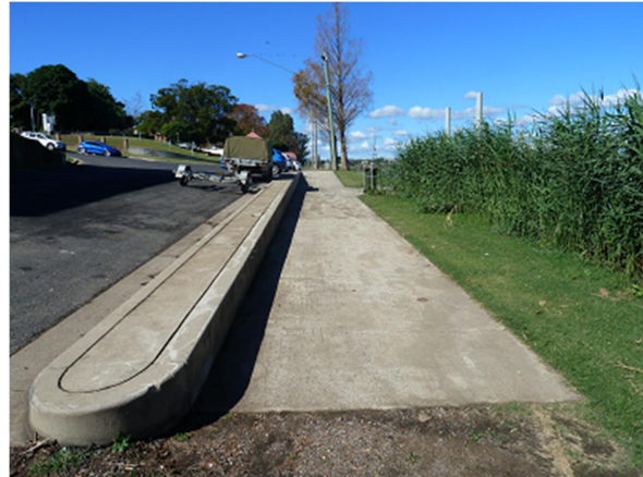
Concrete path, kerbing and road pavement
