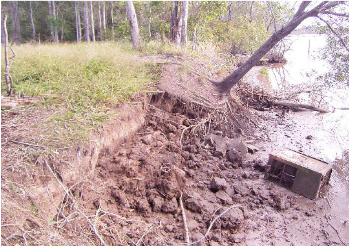
Plate 4. Foreshore erosion (note: left of photo soil compaction and general lack of vegetative structure. Note also rubbish dumping)
