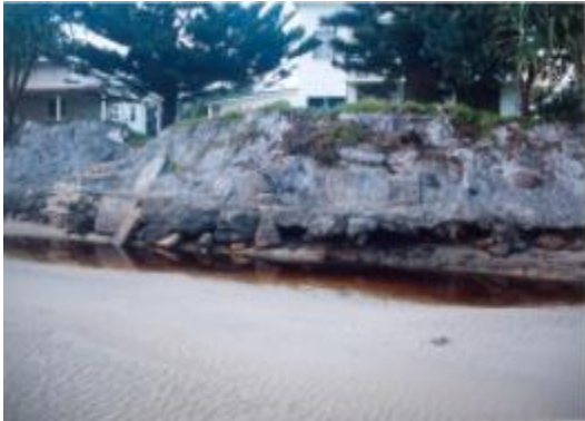
Plate 3 scour at the revetment toe (13/2/2002 source: CVC )
