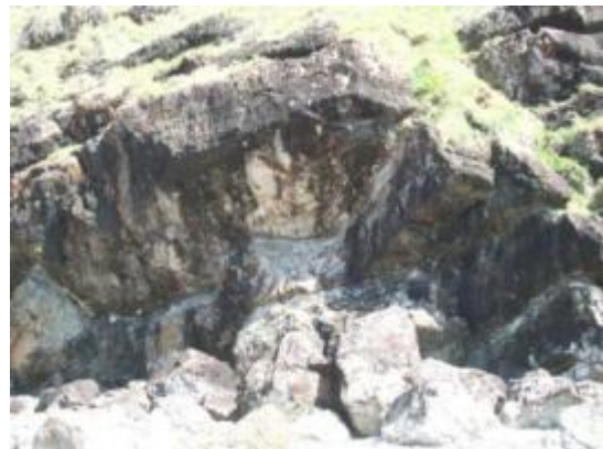
Plate 8 Crest Fretting & Block Toppling Point
