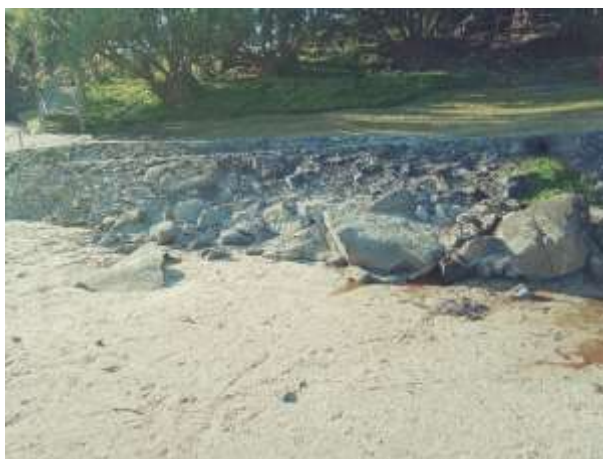
Plate 18: Yamba Main beach rock revetment
