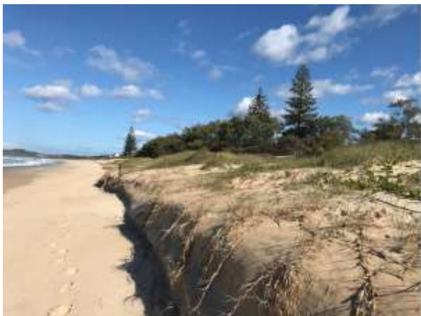
1 – Wooli Beach constructed dune
