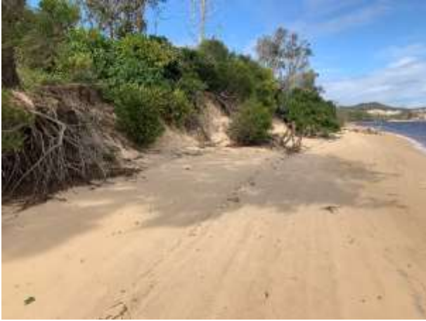
1 - erosion downstream of boat ramp
