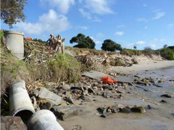
1 - Site after erosion event in 2012
