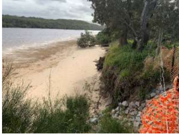
2 - erosion opposite Marine Rescue Tower threatening footpath
