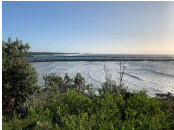
6 – Clarence River entrance breakwaters
