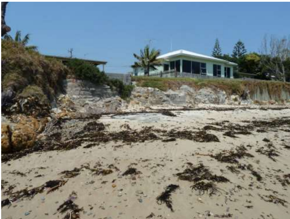
Plate 20: Coastal protection structures at Sandon Village
