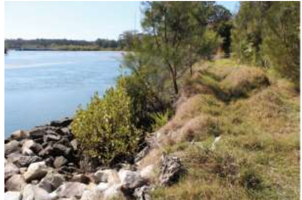
2 - Rock fillets in Romiaka Channel installed in 2008 showing good mangrove recruitment, photo from 2013
