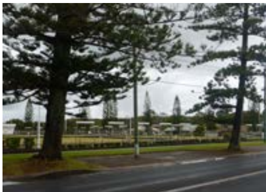
Carpark works have encroached on the roots of the adjacent Araucaria trees. The trees are now suffering stress from root loss. Woolli Street, Yamba
