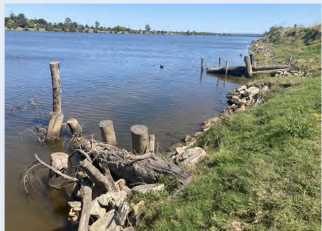
d. large woody debris and rock revetment bank stabilisation
