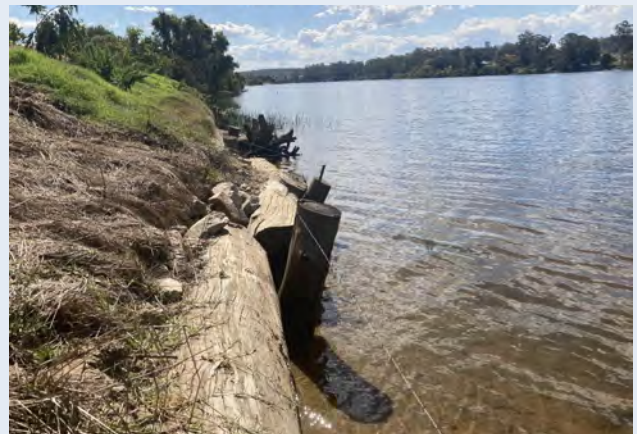
b. large woody debris and rock bank stabilisation structure
