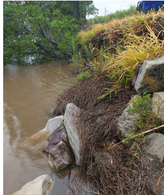
b. Bank erosion and failing rock protection, Goodwood Island
