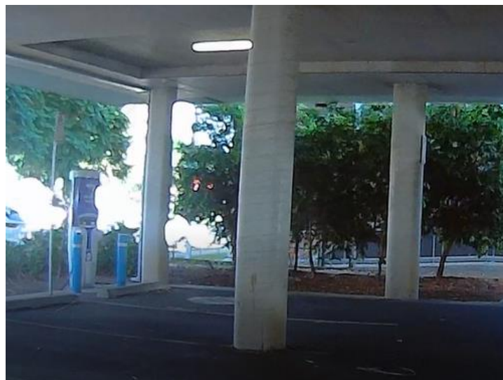
Figure 14: Electric car charging point in the Library carpark
