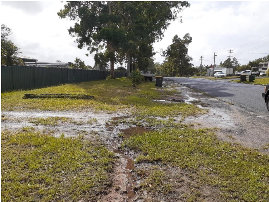
Jubilee Street (facing east) at the boundary of Lot 3 DP1130832
