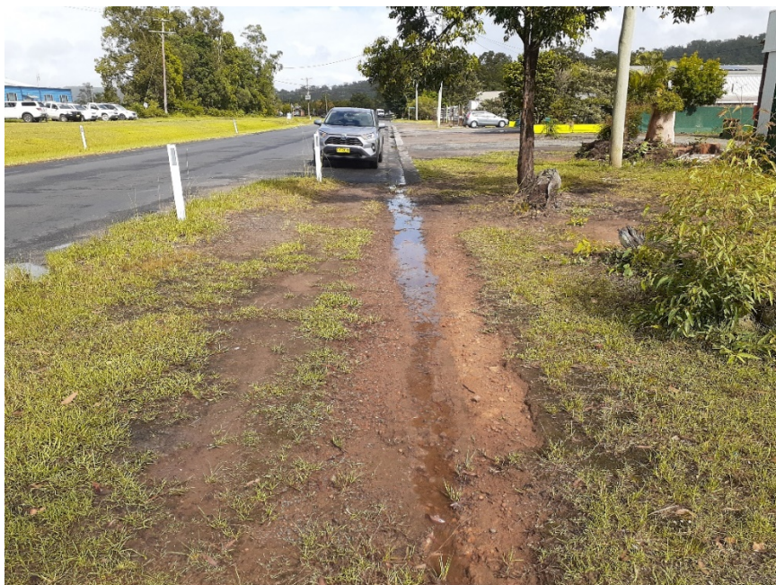
Jubilee Street (facing west) at the boundary of Lot 3 DP1130832
