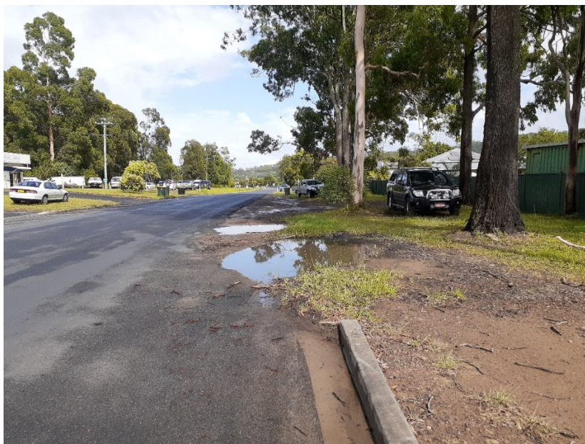
Jubilee Street (facing west) at the boundary of Lot 105 DP877444.
