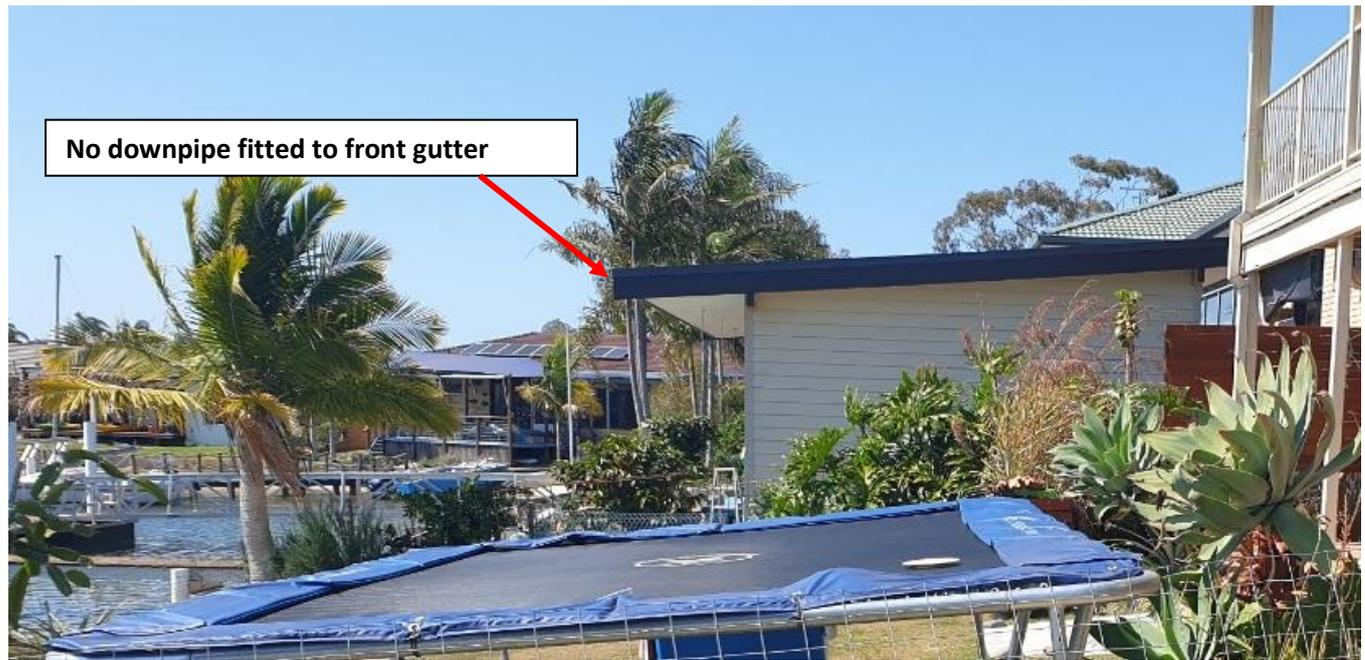
9. Photo taken 5 November 2020 19 Gumnut Road – non-complying roof complete, grey walls clad, downpipe connected to gutter resting along top of non-complying planter box and out over revetment wall into canal for about two months, and non-complying water tank installed (in 900mm setback) with overflow pipe running along ground out over revetment wall to beachfront. 1.8m high non-complying planter box in 900mm setback and 7.5m setback
