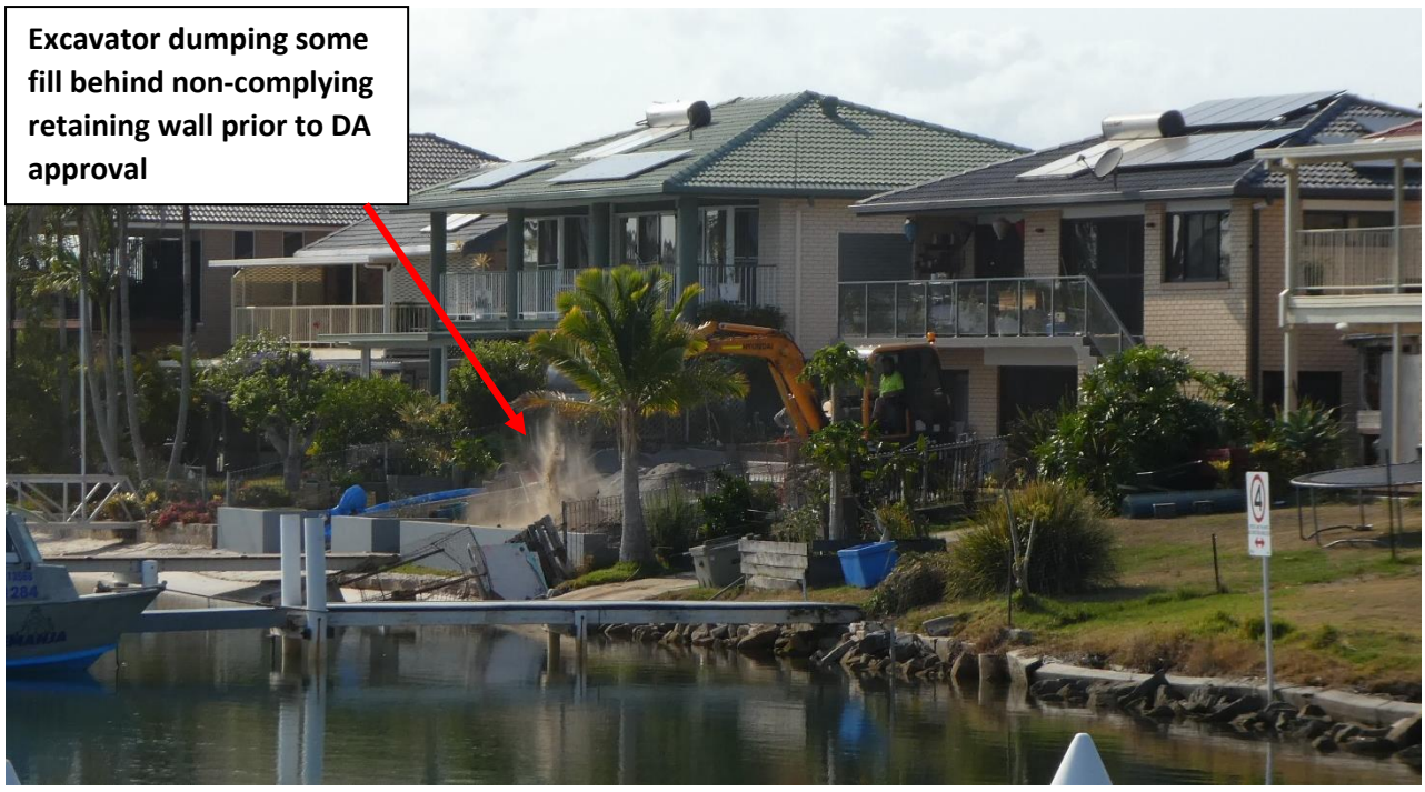
23. Photo taken 19 January 2018 – previous pontoon and jetty at 19 Gumnut Road Yamba – very different structure to new pontoon and jetty installed 30 September 2018.
