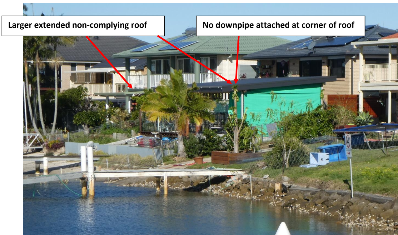
6. Photo taken 16 August 2020 19 Gumnut Road – extended non-complying roof complete on studio - no downpipe visible
