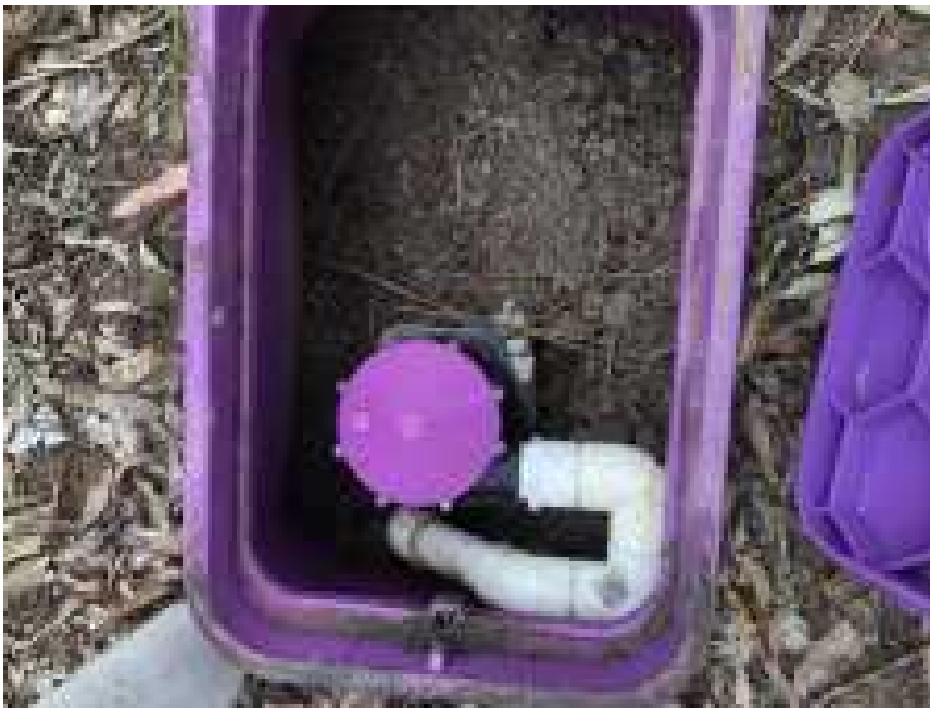
Photograph 9. View of indexing valve.
