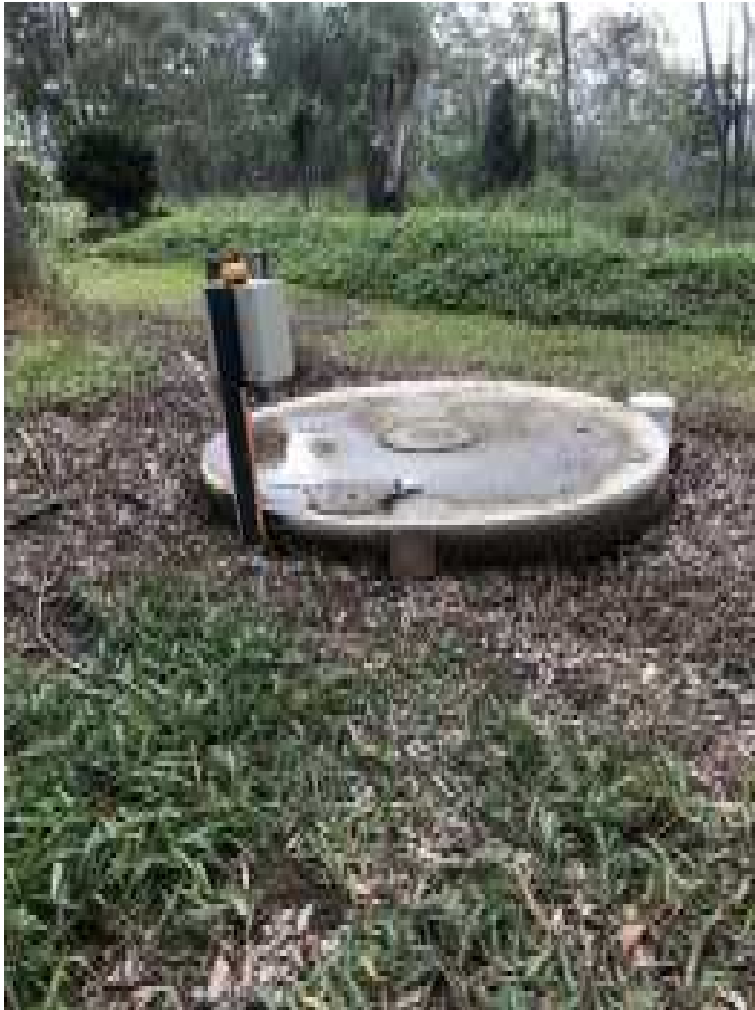
Photograph 7. View of lift well T7 after pond.
