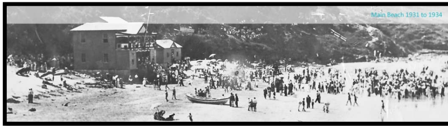
Surf lifesaving clubhouse constructed 1931 (circa 1931-1934)
