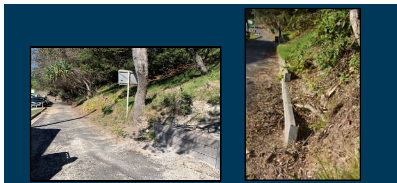
Figure 4.16: Retaining wall behind Yamba Surf Life Saving Clubhouse
