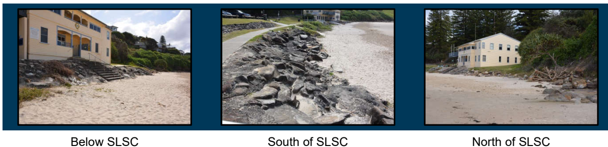
Figure 4.15: Revetment wall and rock protection on Main Beach
