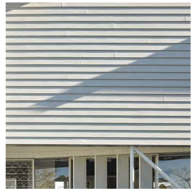
CLD-1 EXTERNAL CLADDING - WEATHERBOARDS - COLOUR AND MATERIAL REFLECTS THE EXISTING MATERIALITY OF THE SURROUNDING BEACH-HOMES IN THE AREA
