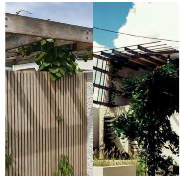
TRELLIS STRUCTURE GROUND FLOOR - SOFTENS EDGE TREATMENT BETWEEN ROAD AND TOWNHOUSES - ALLOWS FOR CLIMBER FLORA STRUCTURE - PROVIDES PRIVACY AND DAPPLED LIGHT
