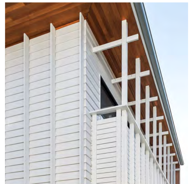
CLD-3 UPPER LOWER FLOOR FEATURE CLADDING - EXPRESSED 'STUDS' OVER CLADDING - PROVIDES ARTICULATION TO SELECTED SECTIONS OF FACADE - TEXTURE AND MATERIAL REMINISCENT OF LIGHTWEIGHT ARCHITECTURE AND COASTAL FLORA
