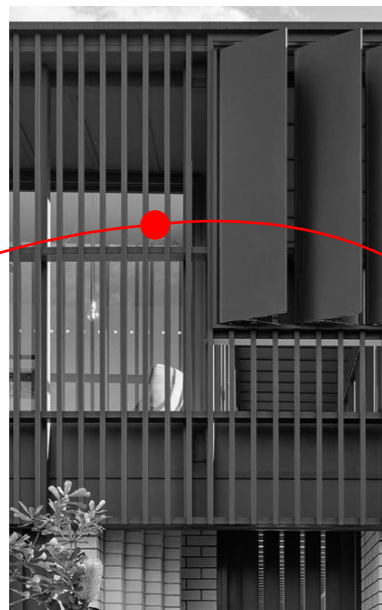
BAL 1 & SCR-2 UPPER FLOOR SCREENS - METAL BATTENS SCREENS - PROVIDE PRIVACY AND FILTER LIGHT - ADD ARTICULATION TO FACADE
