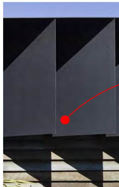
SCR-1 UPPER FLOOR WINDOW BLADES - FIXED SOLID SCREENS - PROVIDE PRIVACY - ADD ARTICULATION TO FACADE - COLOUR VARIETY TO PROVIDE IDENTITY
