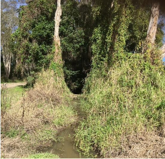
Drains on Schwonberg Street.
