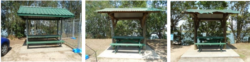
Figure 3.5: Picnic Shelters (South to North)
