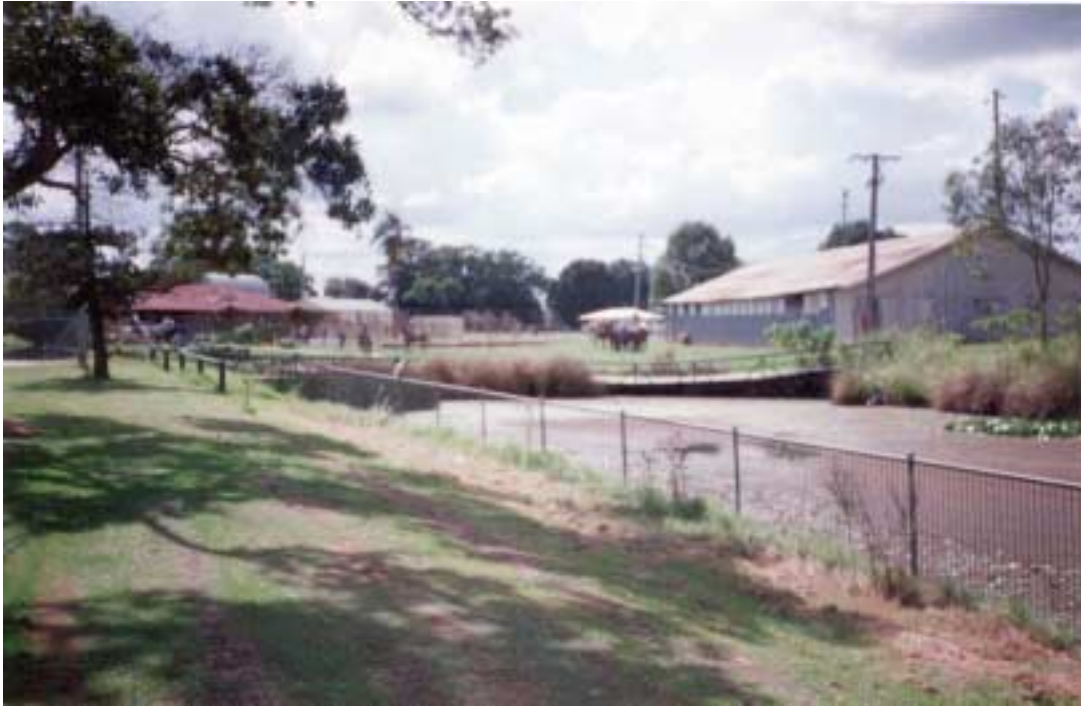
Plate 5 - Safety issues raised include inadequate fencing and structures
