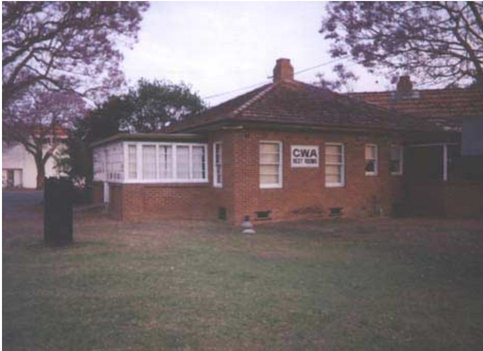
Plate 11: The existing CWA restrooms - there is longer term potential for a visitor refreshment / café facility in conjunction with community groups.
