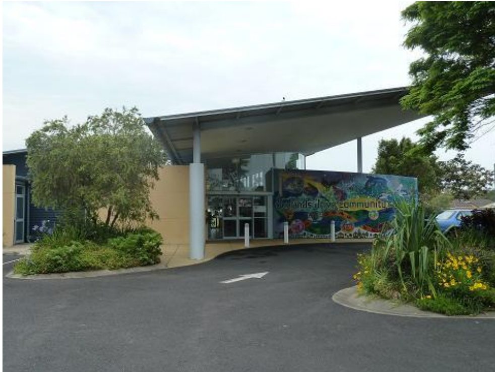
Figure 1.2: Existing Community Centre
