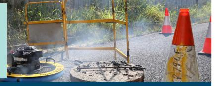
Earlier this year, we completed a smoke detection program in priority areas of the Clarence Valley's sewer network. This procedure involved blowing smoke into sewers at strategic points, with escaping smoke indicating faults. Underground leaks were identified, as well as residential stormwater drains illegally connected to sewers, which put unnecessary pressure on our sewage treatment plants following rainfall.
