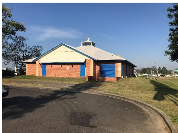
Looking east at the tourist building the filled section can be seen on the right (south).
