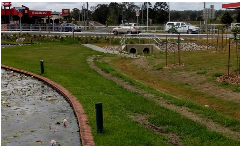
Council Stormwater Drainage
