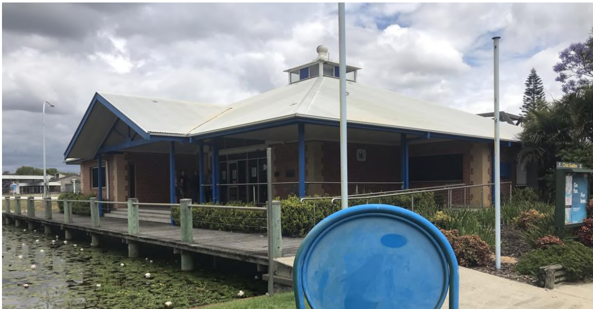
Existing Building on the site
