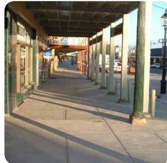
Traditional concrete paving in Coldstream Street
