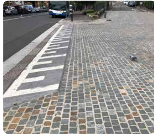
Cobbled vehicular threshold on River Street
