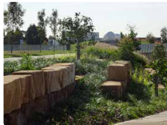
Sandstone retaining walls along boat ramp
