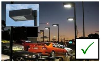
Full cut-off box lights direct light downwards and are cheaper to operate
