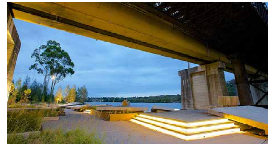
Lighting and seating under the bridge (John Whitton Bridge)
