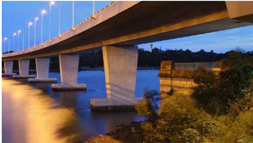
Bridge viewing (Iron Cove Rozelle)
