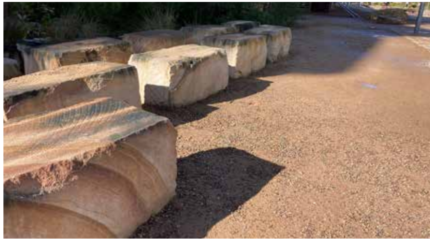
Sandstone blocks to separate road from parklands
