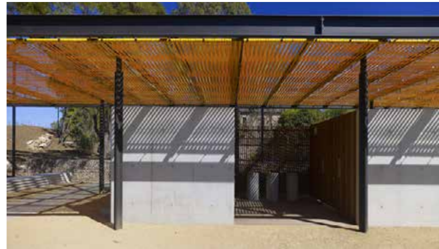
Amenities building (Ballast Point Park)
