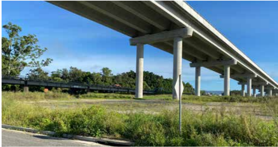
Large expanse underneath new bridge
