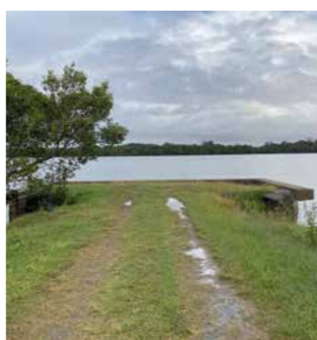
Old public wharf with no heritage interpretation signage
