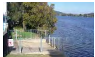
Pumping stations also impede public access along the river bank.
