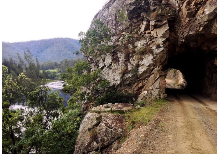
Figure 1: The Old Glen Innes Road through Dalmorton tunnel.
