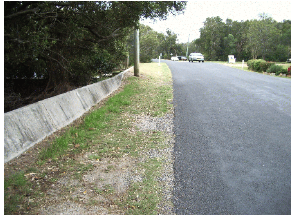
Photo 10: Start of concrete levee opposite The Anchorage Caravan Park
