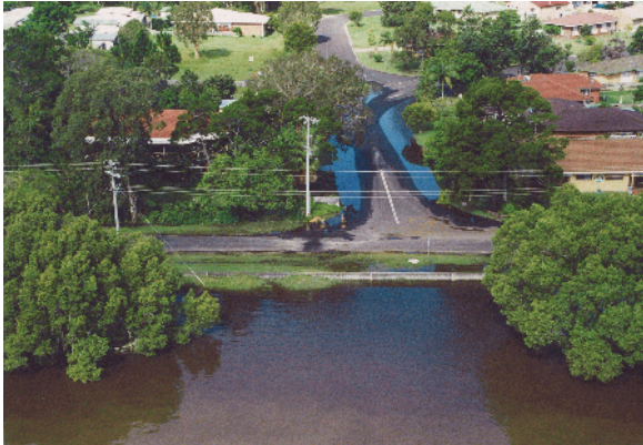
Photo 3: Concrete levee along Marandowie Drive - March 2001 flood
