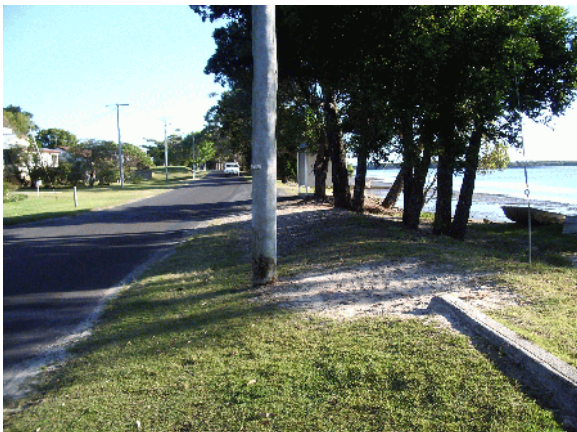
Photo 19: Existing low spots downstream of Marandowie Drive concrete levee
