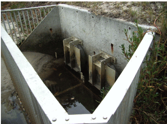
Photo 13: Flap gated culverts within concrete levee system
