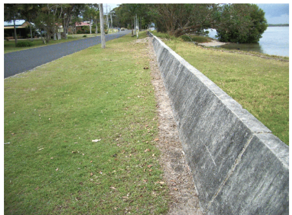
Photo 12: The concrete levee is less than 1 m high
