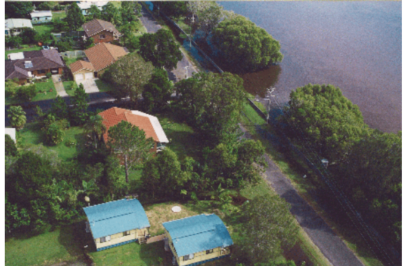
Photo 4: Concrete levee along Marandowie Drive - March 2001 flood
