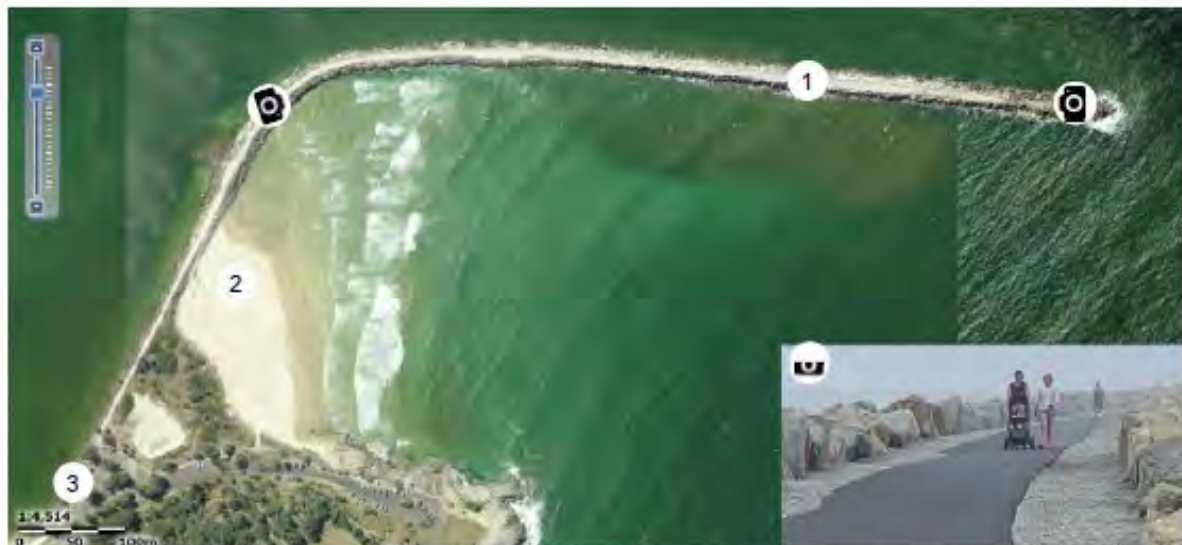
Clarence River Breakwater: (1) the southern breakwater; (2) Turners Beach; (3) interpretative signage acknowledging the engineering heritage of the Port of Clarence breakwater infrastructure. Credit: Six Maps
