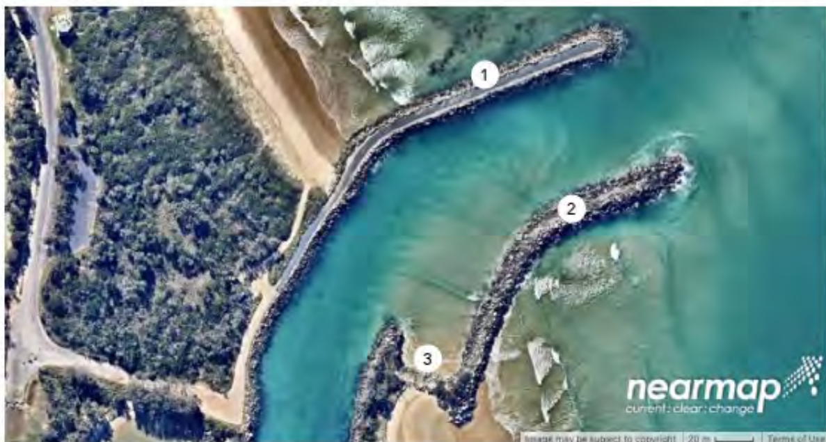
Aerial photo of the Wooli estuary showing (1) northern breakwater; (2) southern breakwater; (3) wave-trap beach
