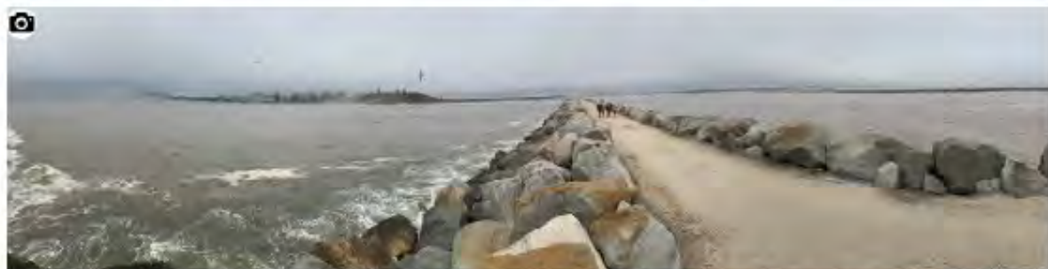
The view back to land from the end of the Clarence River southern breakwater provides a unique perspective as sea birds arc and dive for fish. The first two-thirds of the breakwater has a smooth, tar-finished trafficable surface and the last third is a coarser gravel.
