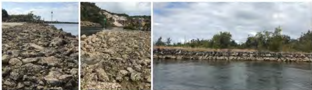
Wooli breakwater rubble has been colonised by oysters to create a valuable oyster reef habitat Credit: Charlie Jenkins
