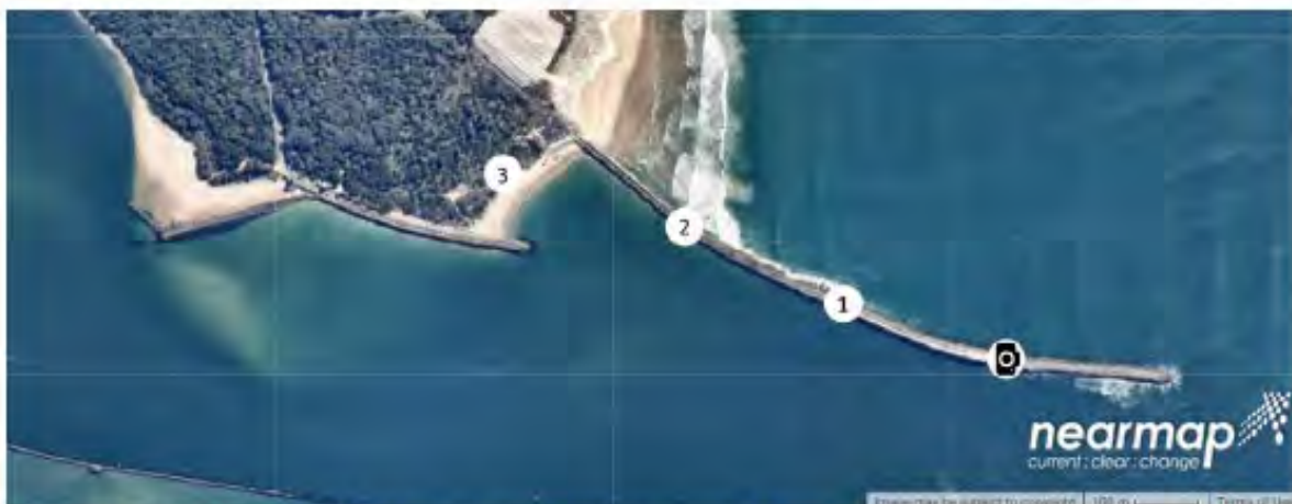
Clarence Northern breakwater, showing the (1) northern breakwater; (2) Shipwreck HMAS Waree; (3) mullet haul beach Credit: nearmap
