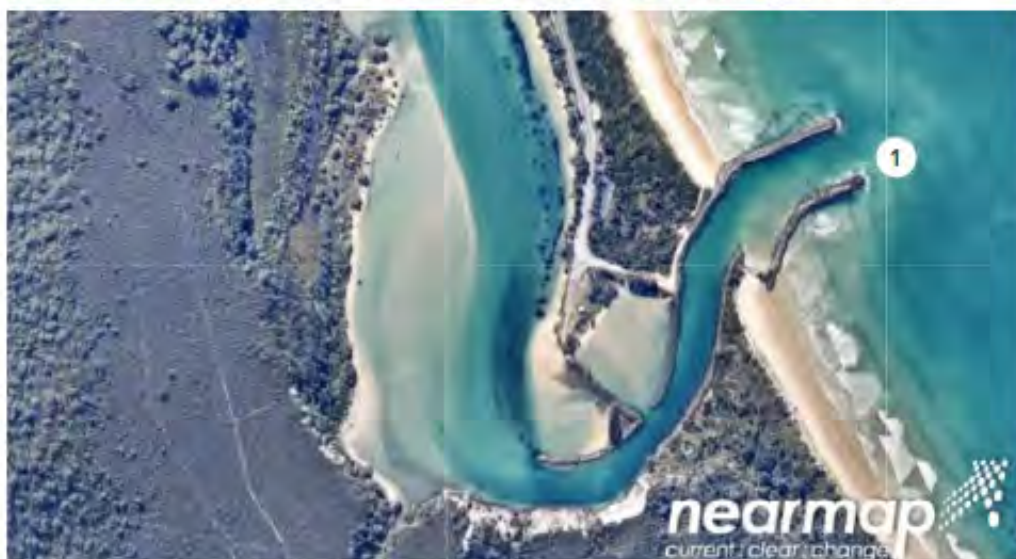
The trained entrance of the Wooli River estuary showing (1) the southern breakwater, the wave-trap beach and the lack of access to the southern breakwater Credit: nearmap
