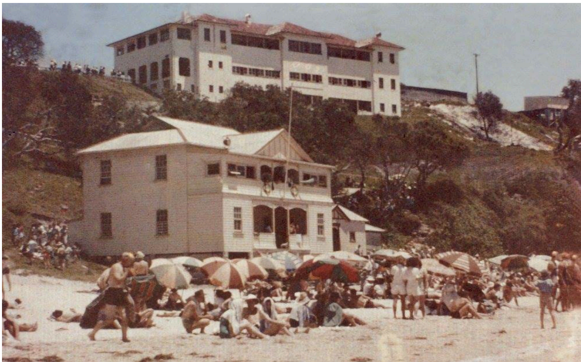
Surf life saving club and Pacific Hotel, photograph taken between 1950 and 1954, prior to slope failure
