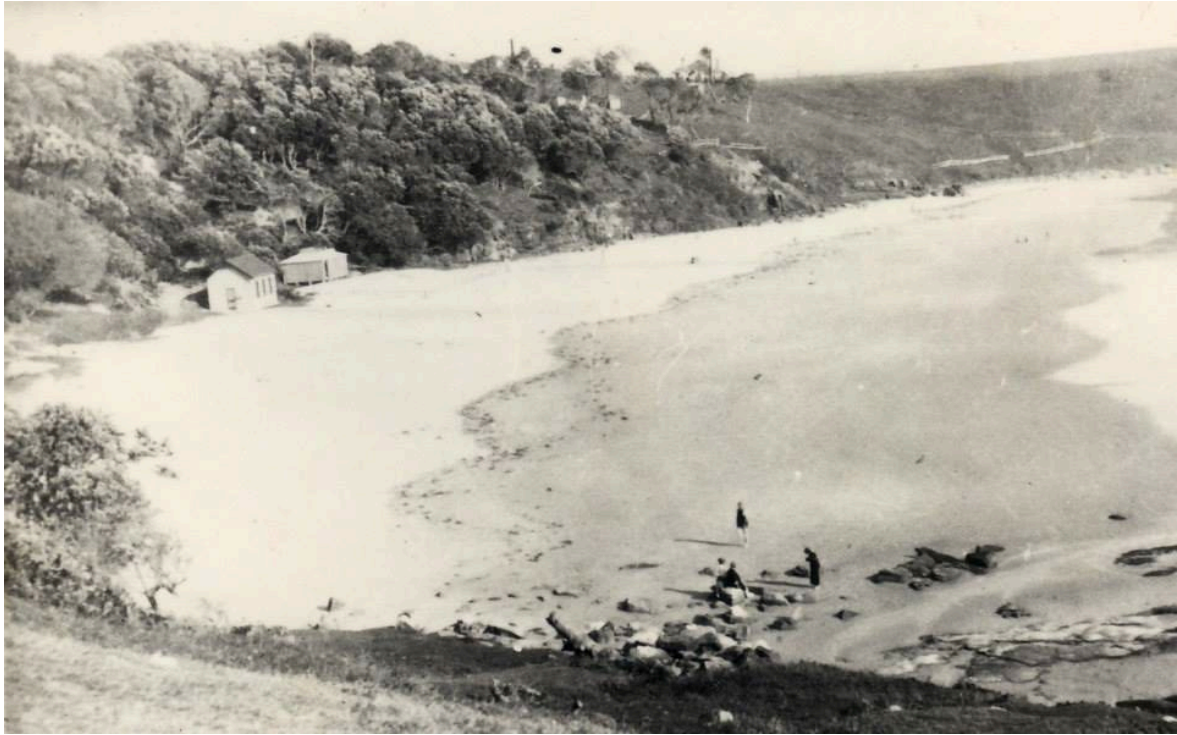
Main Beach circa 1910, looking towards where the Pacific Hotel would be constructed
