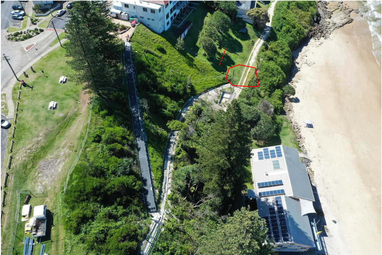
Figure 3-2 Drone imagery of Zig Zag path (taken 10 Feb 2022), an area of land sliding occurred in about the area of red polygon, with tension cracks below the Pacific Hotel shown by red dashed lines. Additional scour and tension cracks affected the road leading to the SLSC (below the photograph above)
