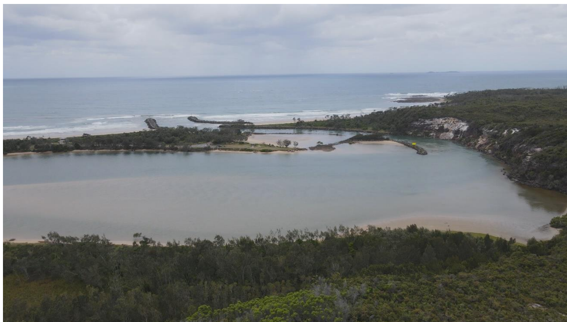
Figure 6-5: Wooli Wooli River entrance, showing training walls
