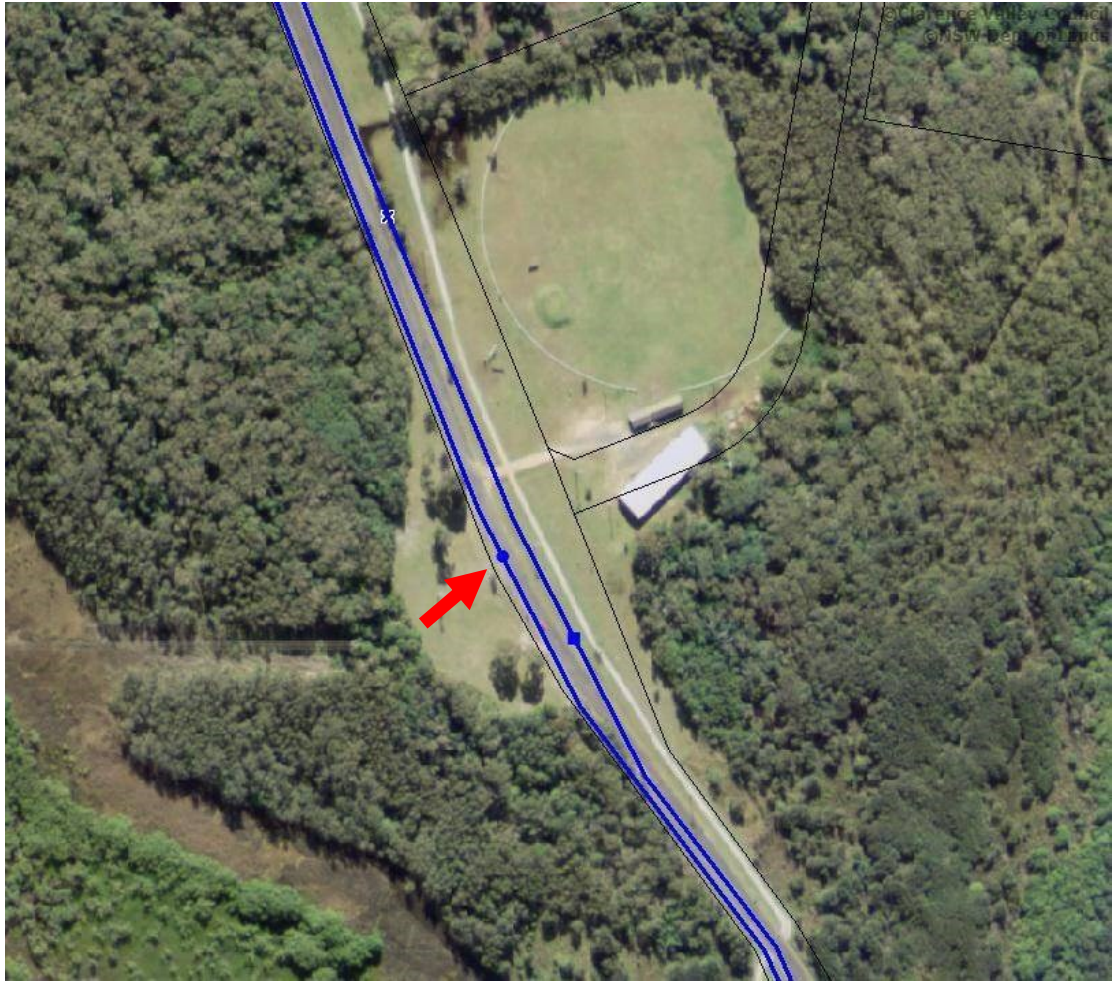
Hydrant 5. Wooli (Sports ground entrance)
