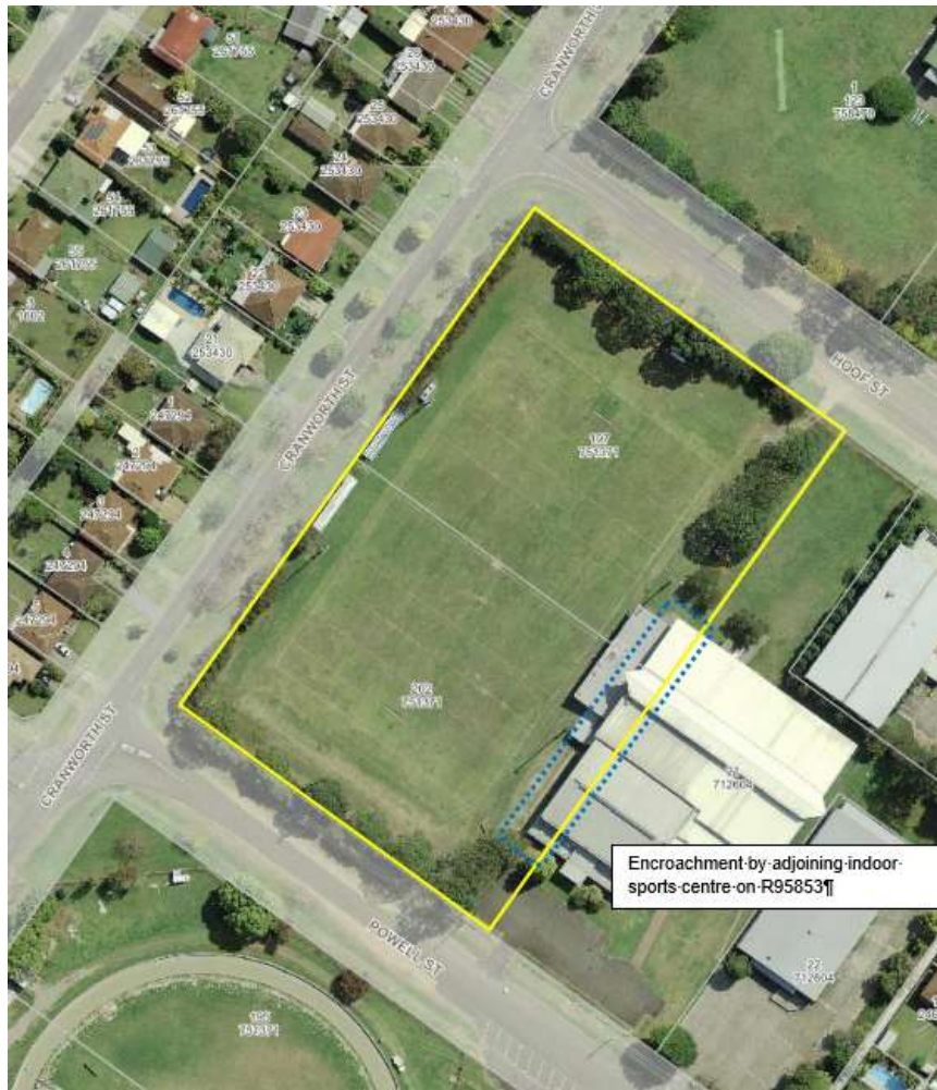
Figure 3 Encroachment of Grafton Sports Complex (on Lots 127 and 202 DP 751371 prior to subdivision)
